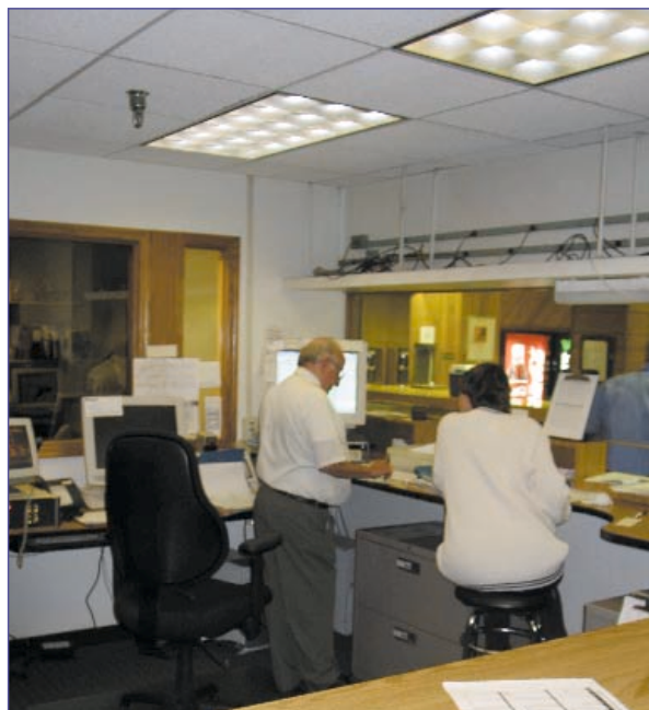
Dimmable fixtures in the dispatch room allow employees the flexibility to set light levels to their comfort.
